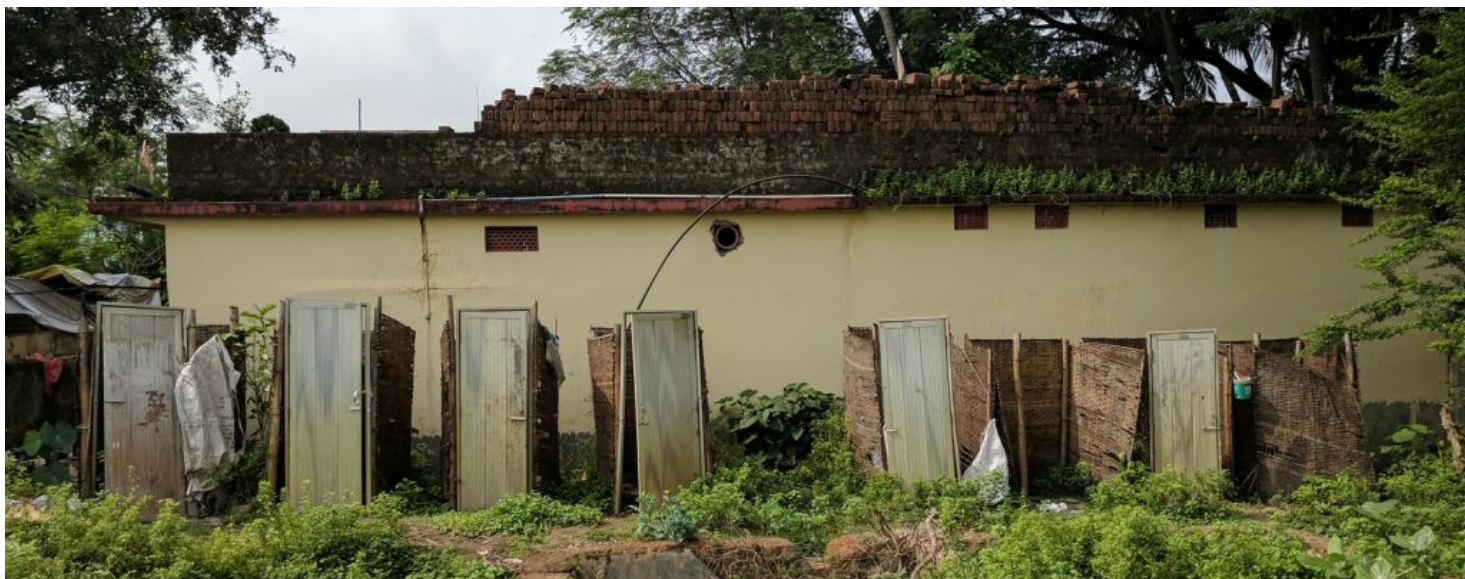
The temporary public toilet for the Macchua Bazaar neighbourhood in Cuttack (a Project Sammaan toilet is under construction nearby). Credit: Gautam Patel
