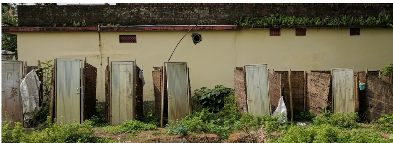
Bottom The temporary public toilet for the Macchua Bazaar neighbourhood in Cuttack (a Project Sammaan toilet is under construction nearby). Credit: Gautam Patel
