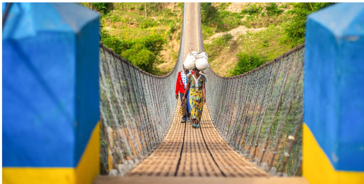
The Gahira Bridge in Rwanda. Photo Credit: Robb Hohmann, Fika
